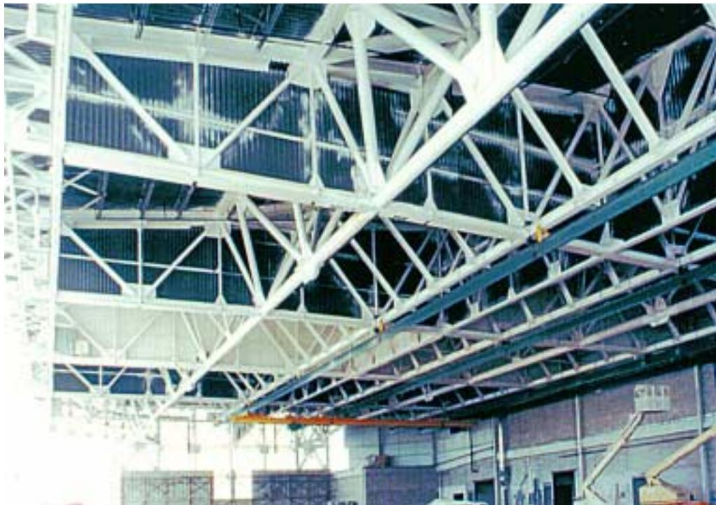
are located through the facility. To enhance flexibility and reduce space, upward acting fabric hangar doors were used requiring special structural details.
